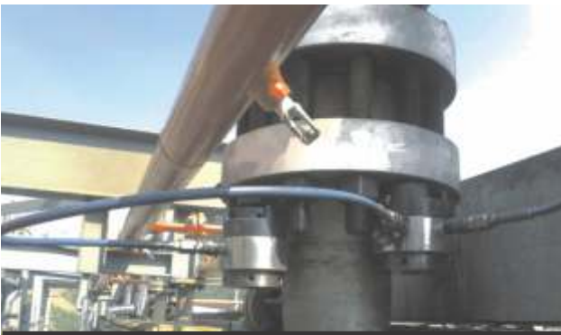
ACCURATE TENSIONING SERVICES
